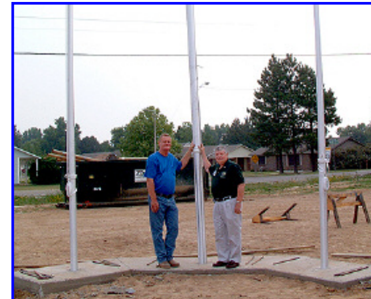
Terry Bailey (left) of Ramsons Construction and Robert Wilford "hold up" the center flag pole of the new flag monument in front of the CRDC administration building. Bailey was instrumental in making sure all facets of construction were on schedule and of the utmost quality.
